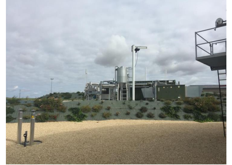
Anaerobic digestion plant with biomethane upgrading and injection equipment at Site 2
