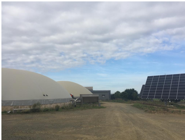
Figure 2 Anaerobic digestion plant and solar panels at Site 1
